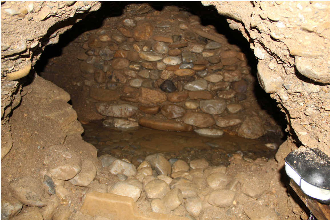
In the Tunnels
